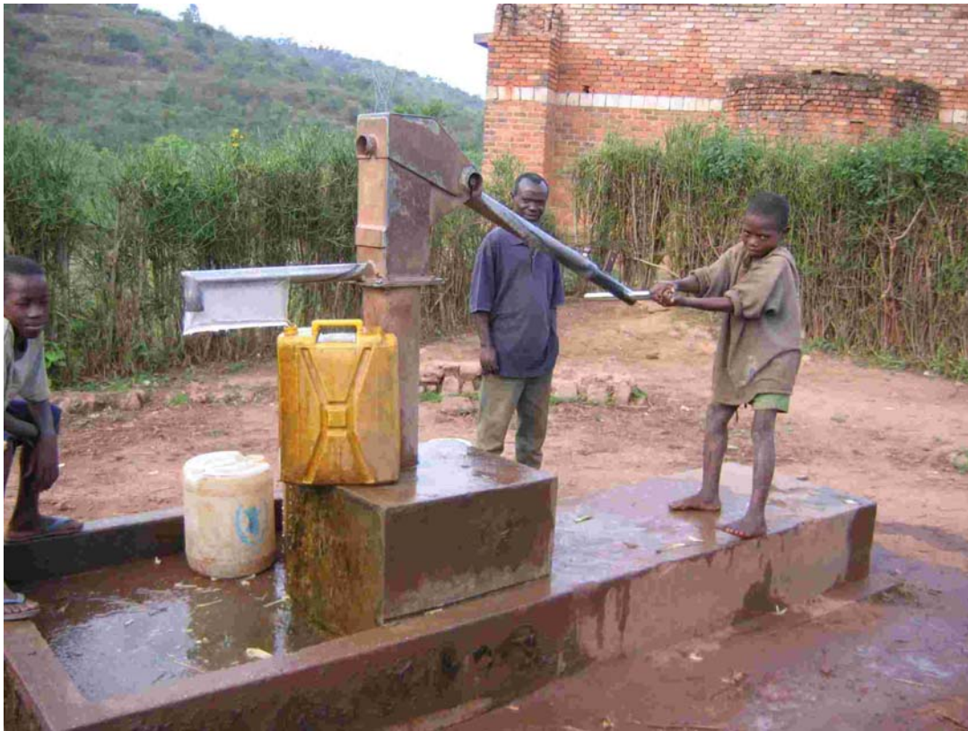
Figure 8. Borehole operated with a hand pump supplies water to a village near Akagera National Park, Rwanda.
