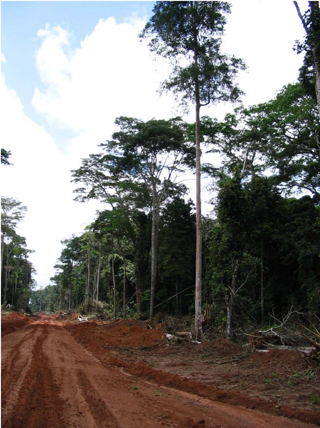
Figure 10. A logging road in the CIB concession in Congo
