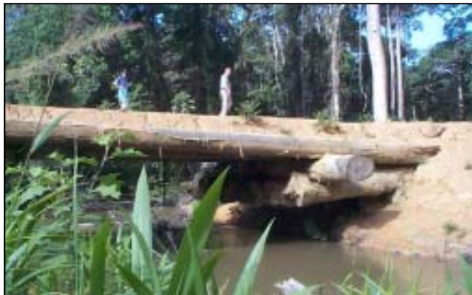
Photo 8. Log bridge in the hilly terrain of the SBL concession.
