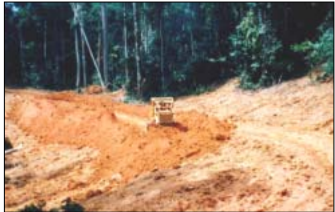
Photo 20. Bulldozer constructing a logging road on the SBL concession.
