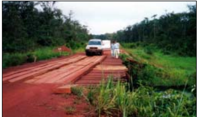
Photo 7. Log bridge at CIB. The approaches to the bridge have been built up as dikes in order to cross an extensive area of swamp.
