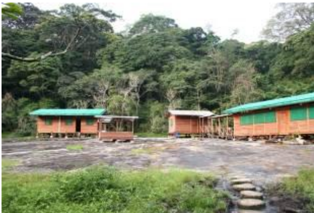
Office, kitchen, dining area
