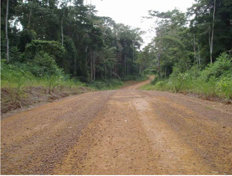
Photo 1-Well maintained Principal Haul Road.
