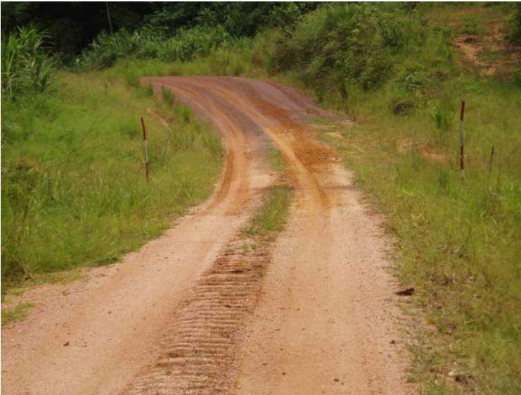
Photo 14- Spot rocking (background) with local laterite rock on a steep grade.
