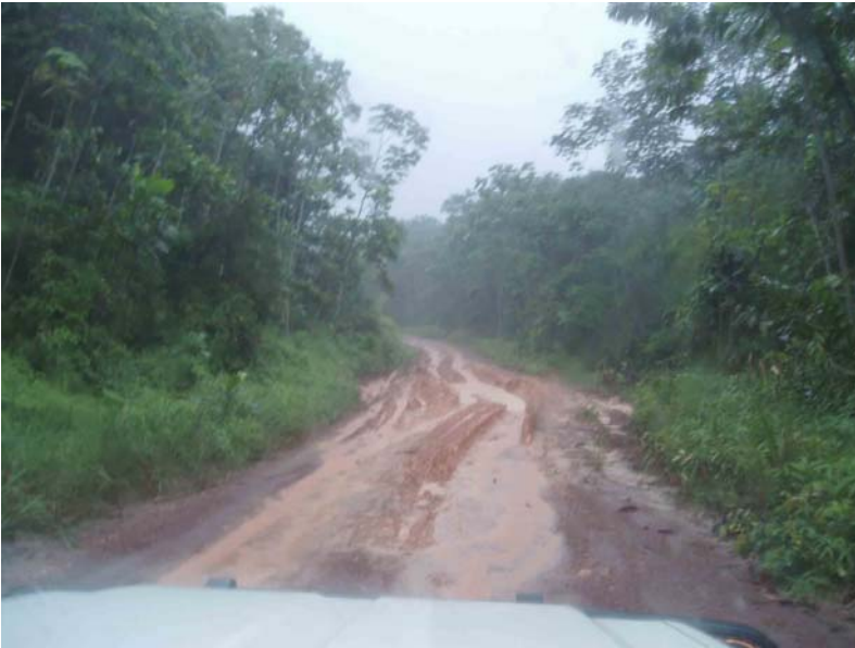
Photo 8- Nearly impassible mud holes when raining (NR 3).
