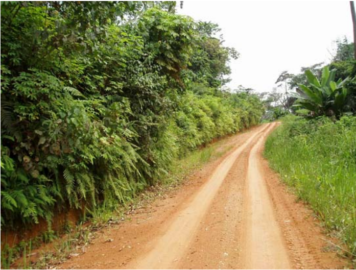
Photo10. Well vegetated stable vertical cut in a clay rich soil.
