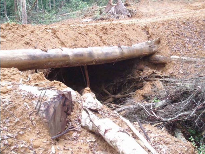
Photo 11- Typical log stringer bridge utilizing locally available logs.
