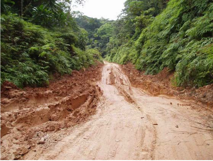
Photo 7- Mud hole in National Road 3 due to lack of Maintenance.
