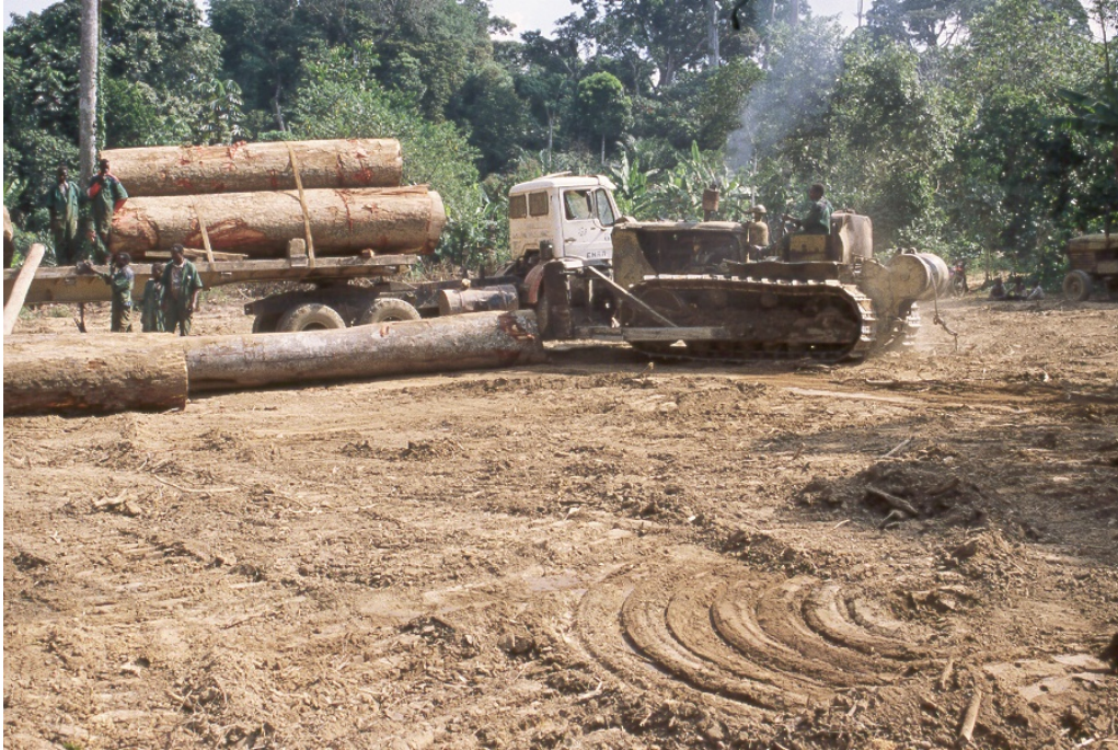
Fig. 5. Loading bay and logs being loaded on a truck in ENRA concession. Log landings, along with logging roads, are the most severely disturbed areas by logging operations.
