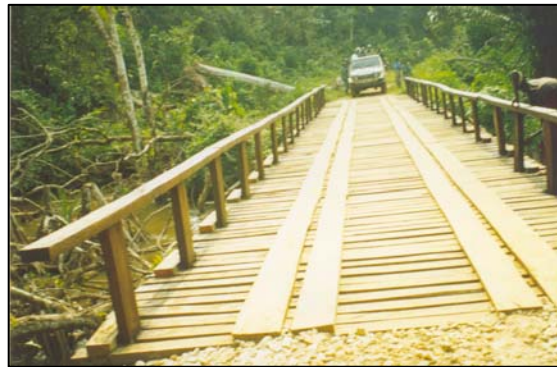
Bridge built as part of road rehabilitation in northeast sector of Maiko National Park. This bridge, built by temporary labor hired from local communities, functions to provide access to the park for ICCN staff, and also provides local farmers access to market.
